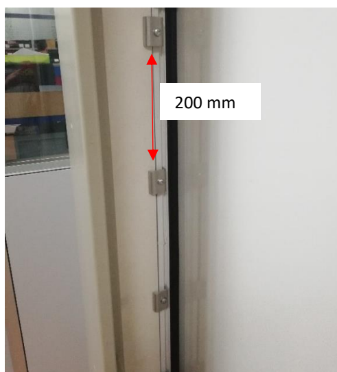
Picture 22 Fixing of the clips on the wall.
