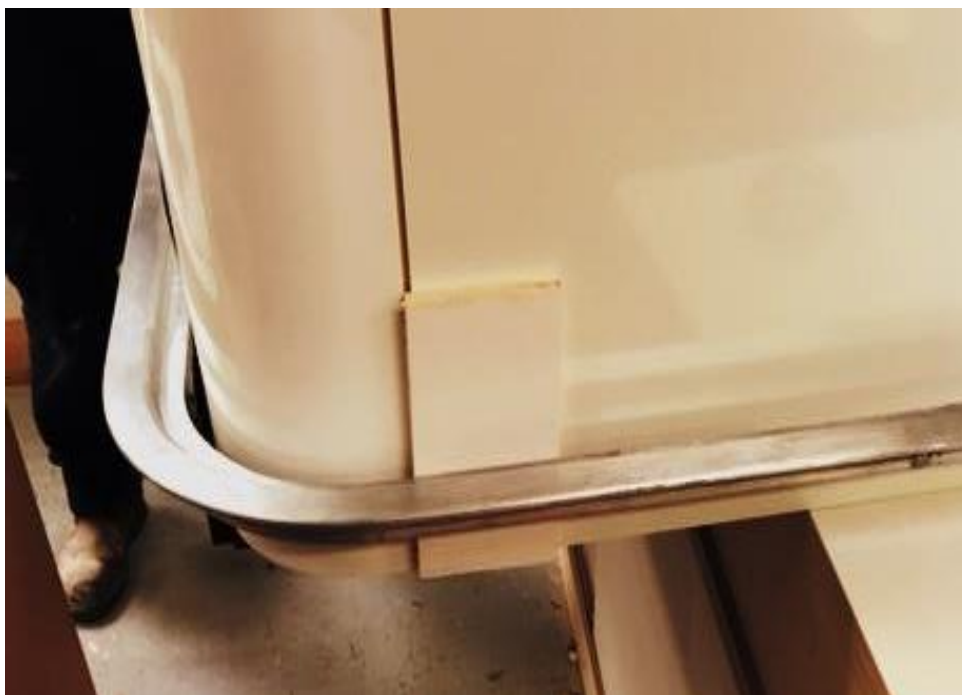
Picture 14 Check the clearance with 13mm spacers.
